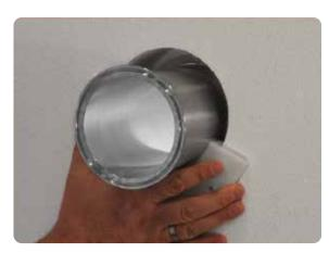
Make sure that the support rings are placed tight and horizontal.
